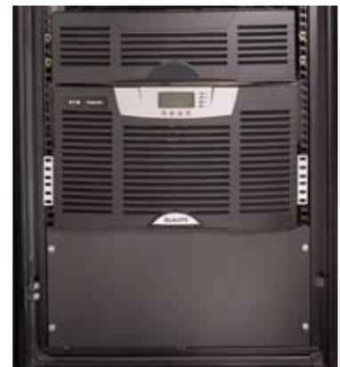
Single Powerware BladeUPS with EBM (12 kW)
